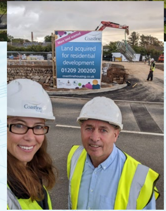
Jo Harley, Development Manager at Coastline Housing, stands with Neil Morton, Classic Builder's Site Manager at Nancegollan, where work has begun on 19 new affordable homes.
